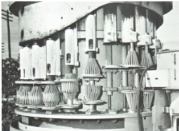
**402X with covers removed.** 24 heads, 20 strokes/480 fruit per minute. Note 20 finger cup with strippers.
