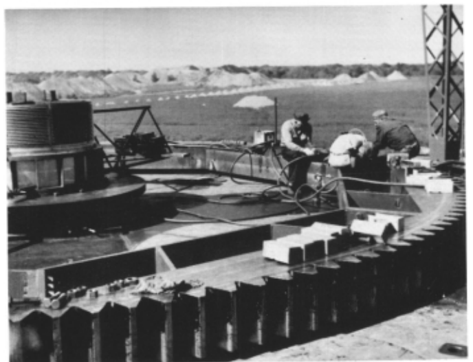
Figure 2. Workmen assemble the huge turret gear.
