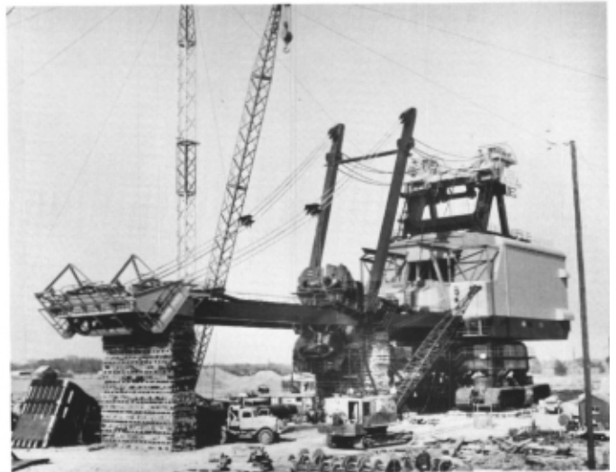
Figure 1. Fifty-two men worked eleven months to assemble Big Brutus.
