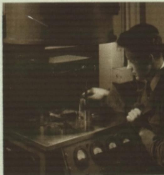
*Aluminum plates were coated with selenium at Battelle using this vacuum system.*
