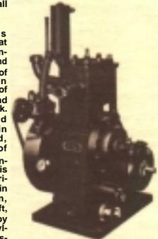
Figure 3—Fixed Compression Engine showing Battery Ignition System, Steam Cooling Condenser, and Water Pump.
