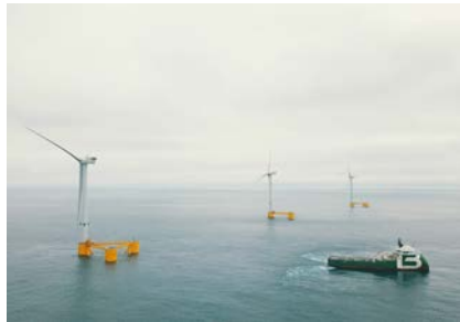
WindFloat Atlantic floating wind farm. Image courtesy of Principle Power
