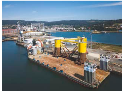
WFA unit being loaded out in the water semi-submersible vessel. Image courtesy of Principle Power
