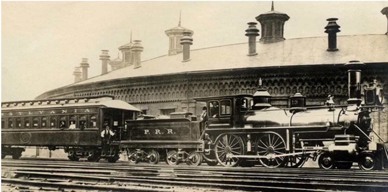
The first locomotive equipped by George Westinghouse with compressed air brakes in 1869 on the Pennsylvania Railroad. The steam driven air pump was installed between the two drive wheels.
